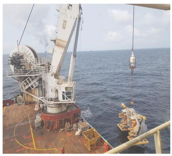
Positioning and Navigation of Construction barges needing anchor monitoring, flexible umbilical pipeline layback positioning and Mattress installation support.
